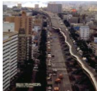
Figure 1. Failure due to soil pile structure interaction (SPSI)
