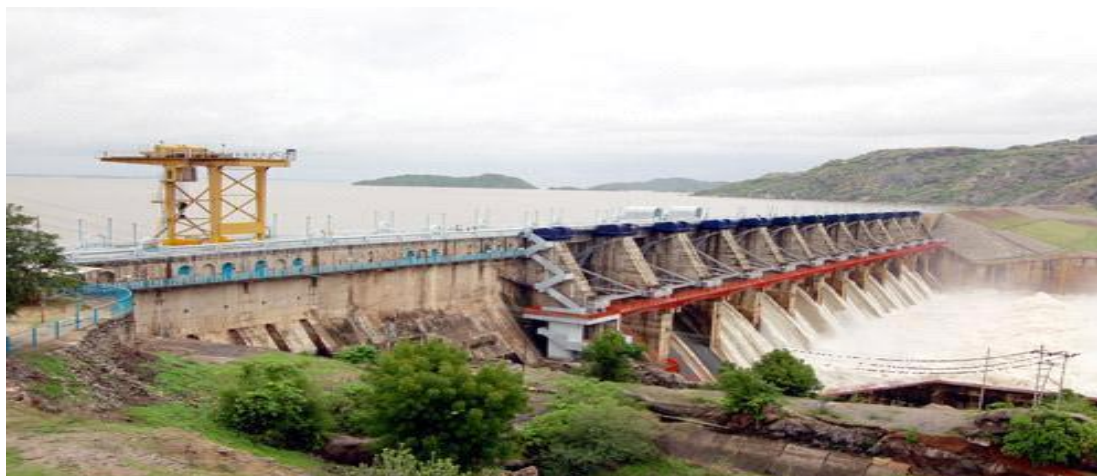
Fig. 3: Image of Dharoi dam
