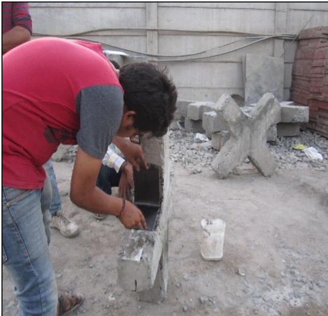
Figure 5. Wrapping of CFRP
