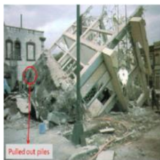
Figure 1. Failure due to soil pile structure interaction (SPSI)
