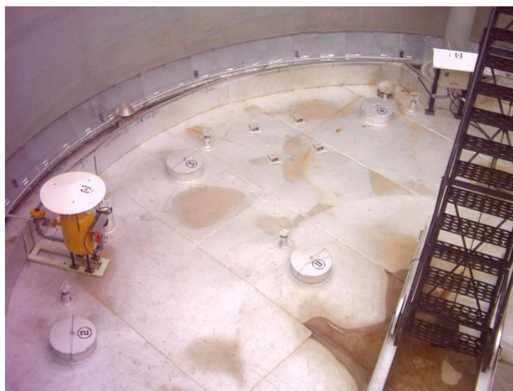
Fig.1 Rim seal fire protection system
