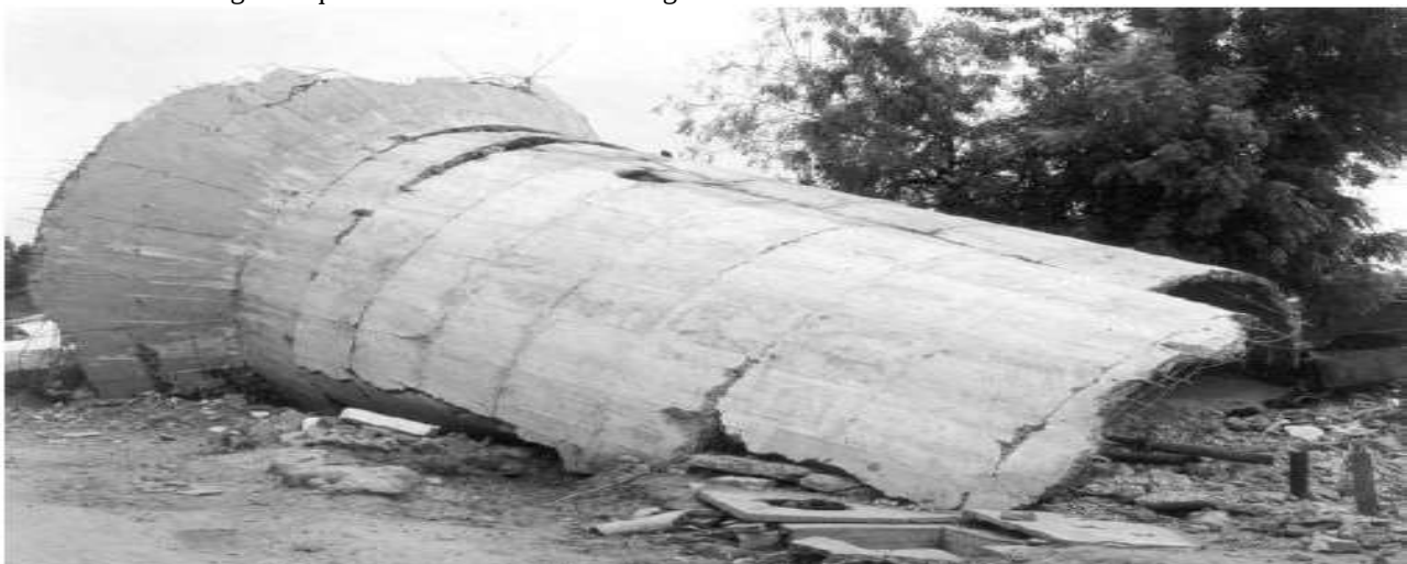
Figure 1. Collapsed 265 KL water tank in Chobari village about 20km from the epicenter. The tank was approximately half full during the earthquake. (Source: - paper presented by Durgesh C. Rai)
