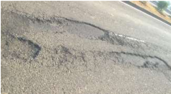
Figure-1 Pothole
