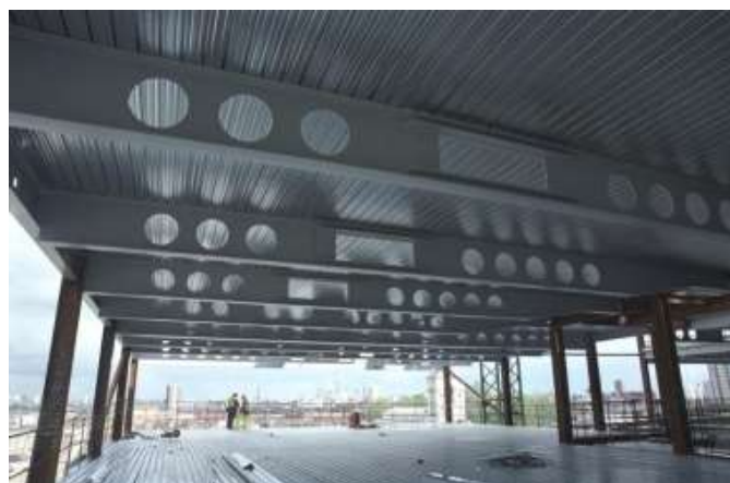
Figure 1 Steel beam with web opening
