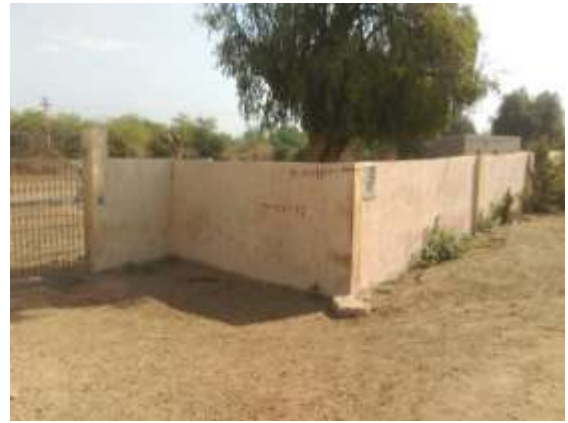
Figure 4. After Pumped out water in Nagala Village
