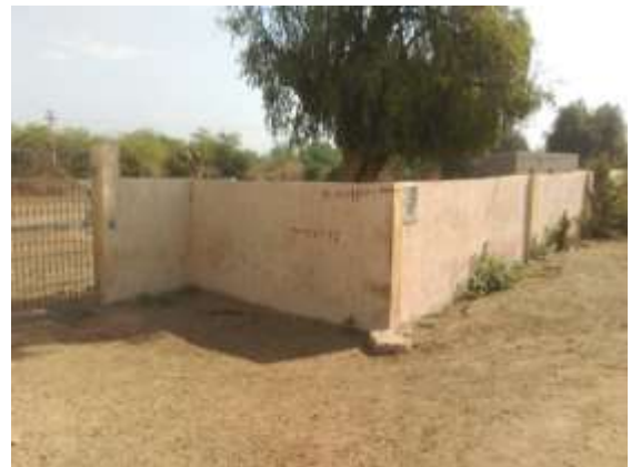
Figure 5. After Pumped out water in Nagala Village
