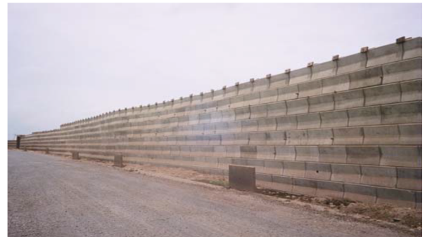
Figure1. RE Wall elevation using Geogrids
