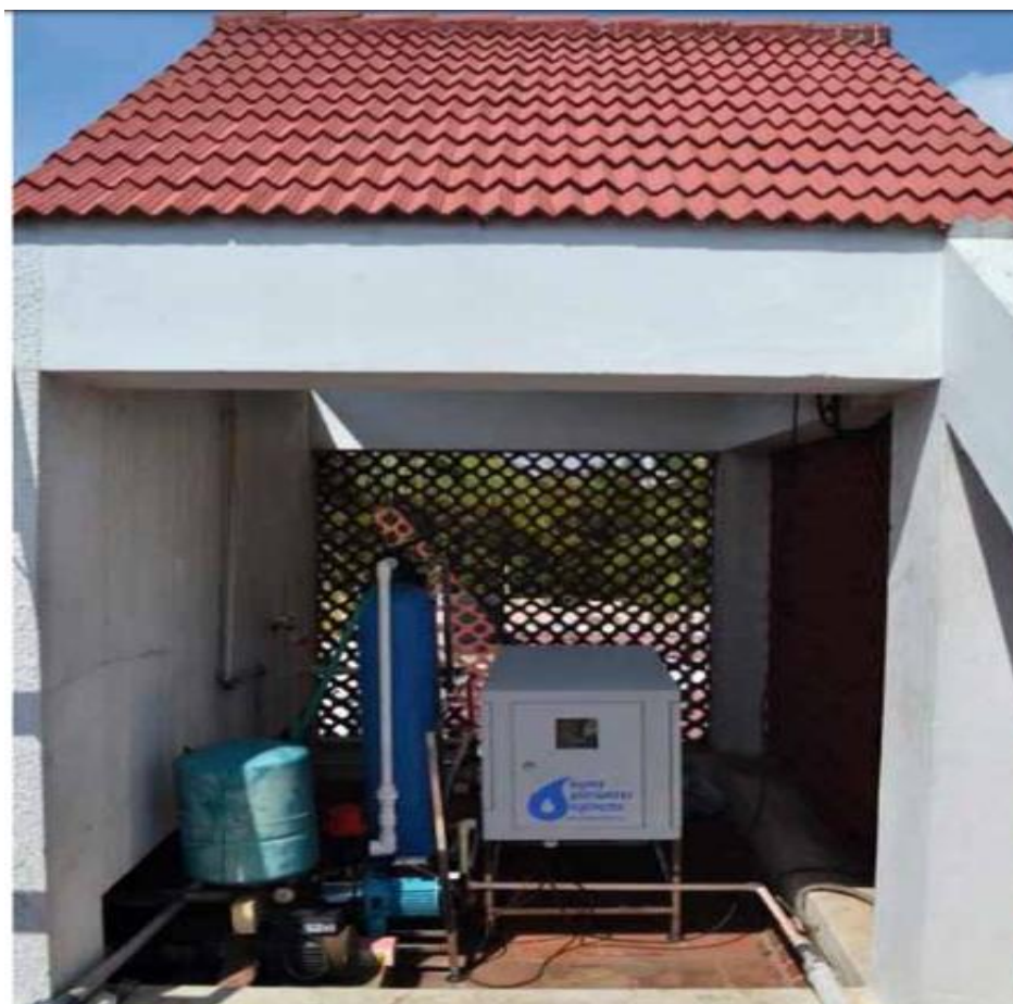
Figure 3: CDI used as a point-of-entry system for treating incoming water for residential homes.
