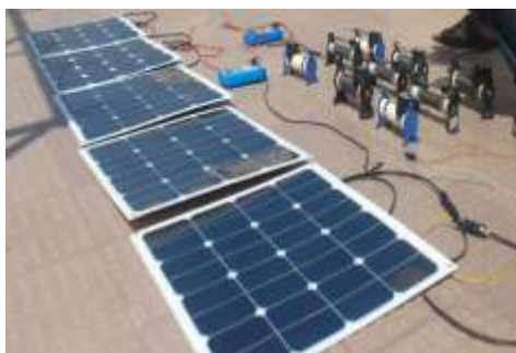
Fig 6: The 50w semi flexible solar panels used
