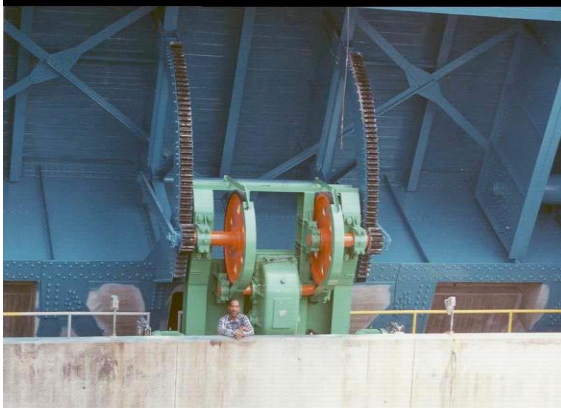
Figure 2. Movable Single Bascule Bridge with the Operating Gearbox Mechanism
