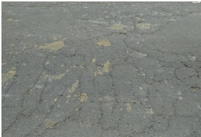
Figure 12 Alligator Crack ( Chainage 10.700 km )
