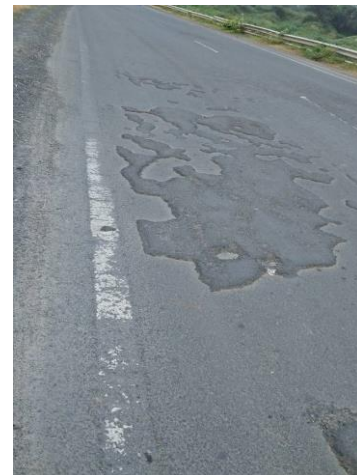
Figure 13 Surface Up Heave ( Chainage 17.200 km )
