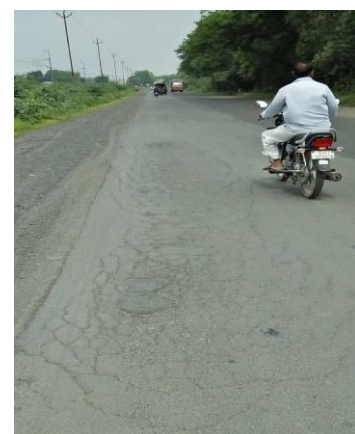
Figure 9 Map Cracking ( Chainage 8.600 km )
