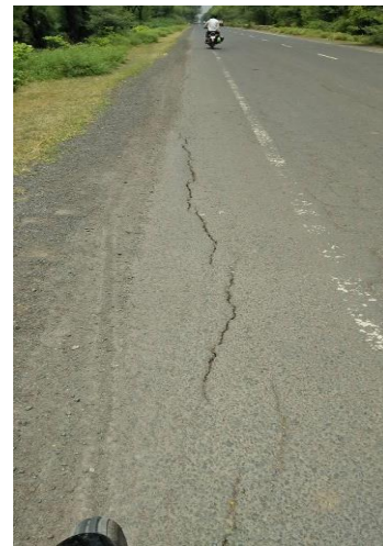
Figure 11 Longitudinal Crack (Chainage 13.700 km )
