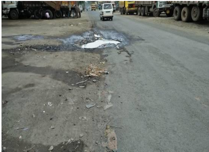
Figure 10 Pot Holes (Chainage 1.200 km )
