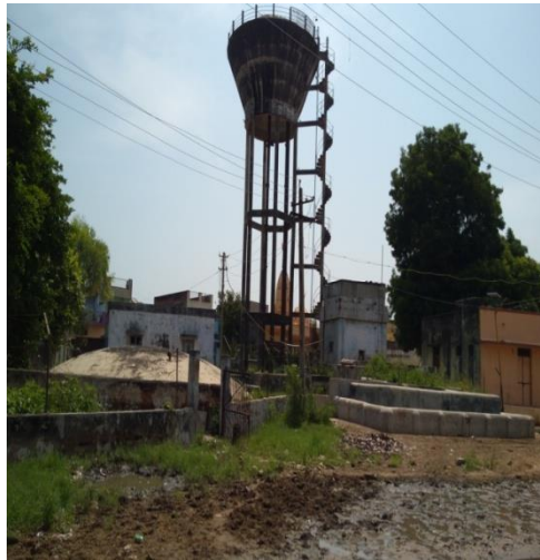
Fig 3:- Elevated storage Tank (1 lakh Litres)
